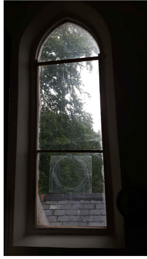
Detail of "temporary" window to be replaced with a new timber framed window glazed with original glass which has been kept in storage.
