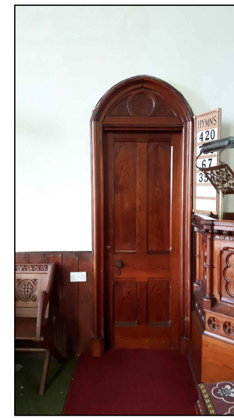
Existing door in chapel to be removed.
